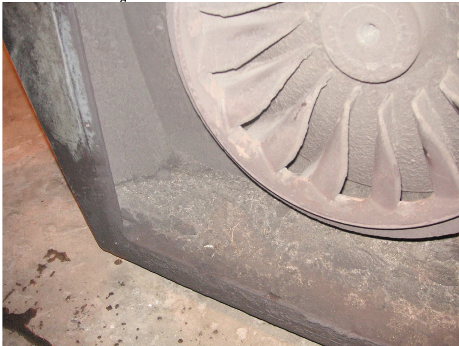
Figure 5: Fan Condition and Contamination
