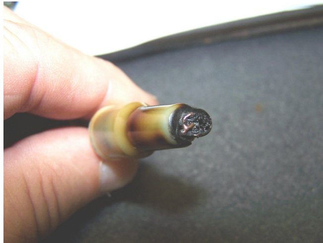
Figure 3: Defective Crimp Connection (a)
