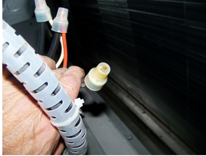
Figure 1: Crimped Connections (1)
