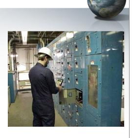
For the system under review, the following potential problems consist of loose connections, worn contacts and failed power factor correction capacitors. Test methods that can be utilized to review the condition of these components include:
