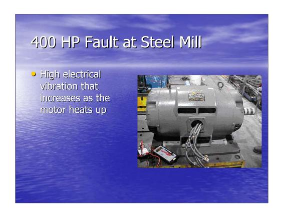
In this first case study, a problem in a 400 horsepower electric motor at a steel mill was identified. This problem had been driving the maintenance and reliability group crazy for about two months. As it was part of a parallel system, this motor was used only as a back-up, which created another problem – an unreliable back up system.
