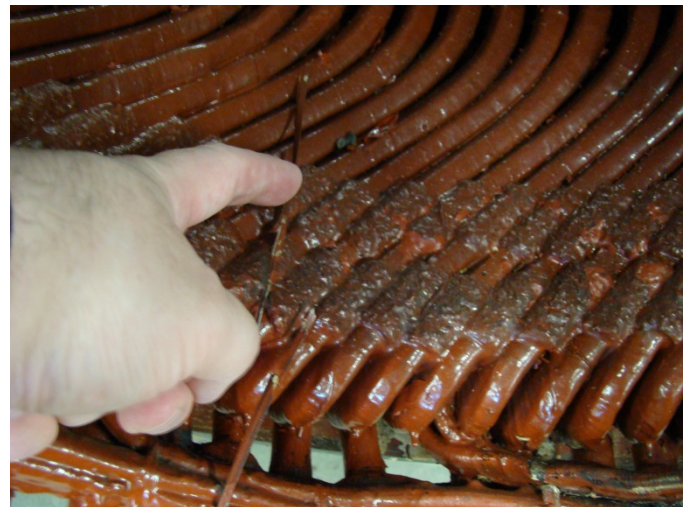
Figure 5: Visual Inspection of Winding
