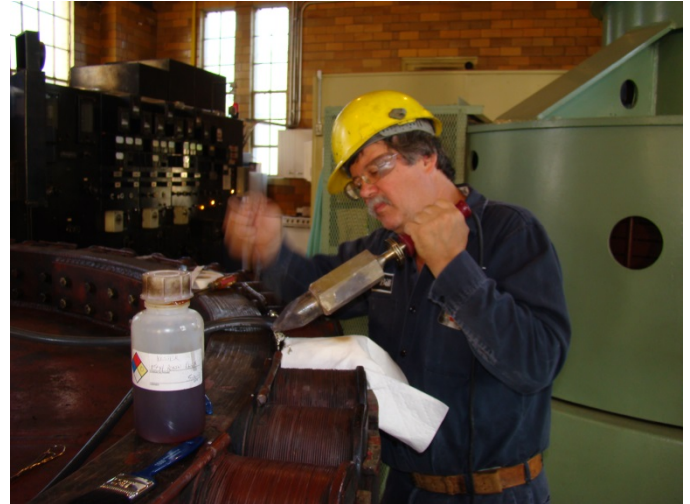
Figure 14: Field Repair of Generator
