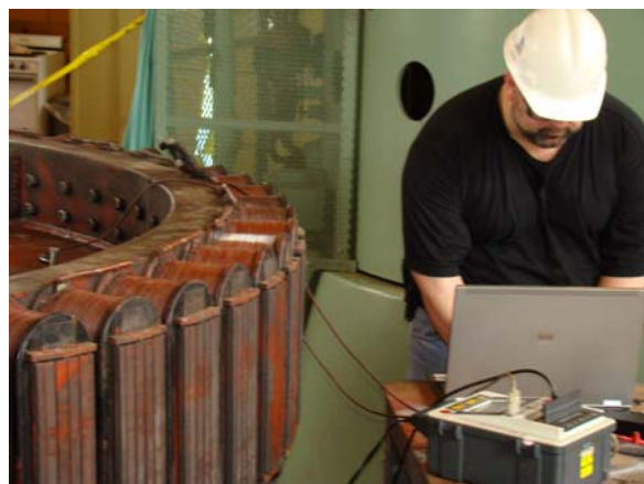
Figure 2. Test Setup for IRP Testing on Rotor
