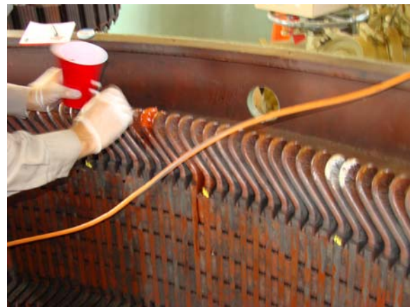
Figure 5. Application of the Weeping Epoxy
