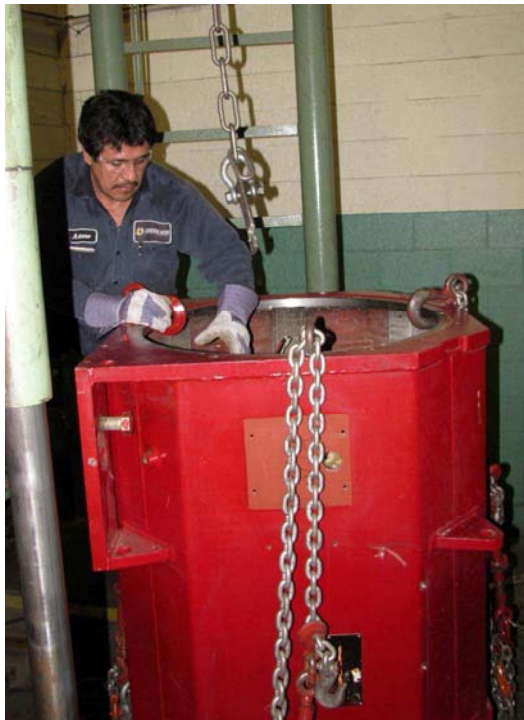
Fig. 2. Stripping Generator Vertically
