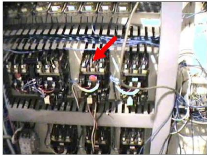
Figure 2: Evaluation of a Loose Bus Connection
