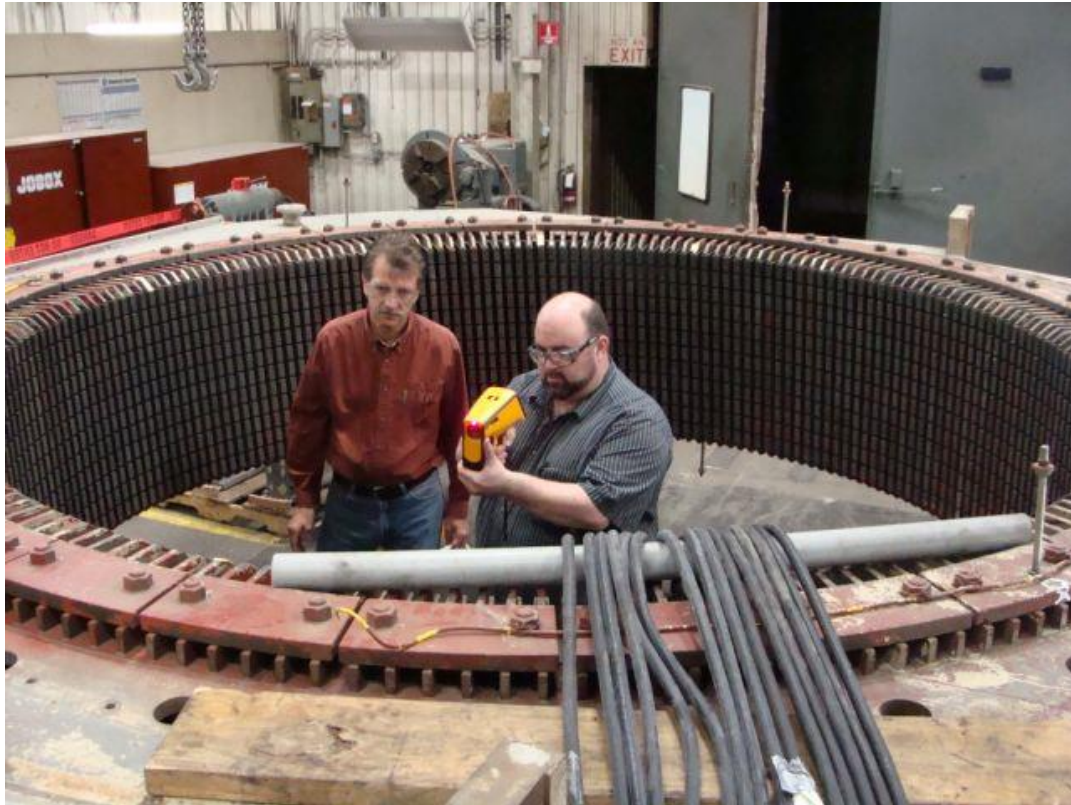
Figure 10: Thermography Performed to Find Shorted Laminations on a Large Stator
