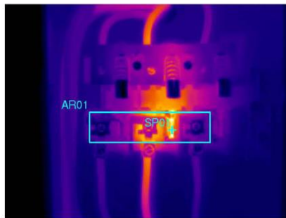
Figure 5: Loose Connection on Switch for Elevator
