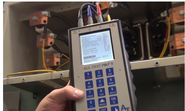
Figure 6: ALL-TEST Pro 5 testing an assembled form-wound stator
