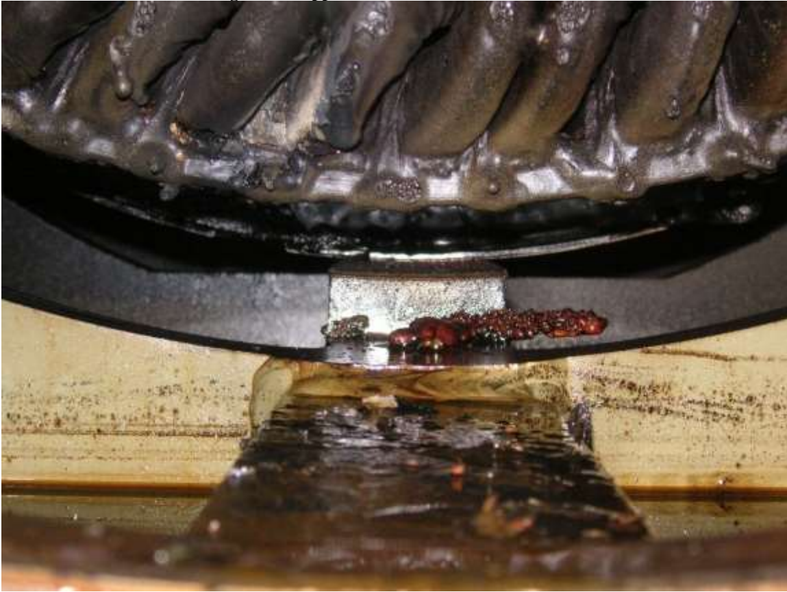
Figure 4: Copper from Louis Allis Coil Failure
